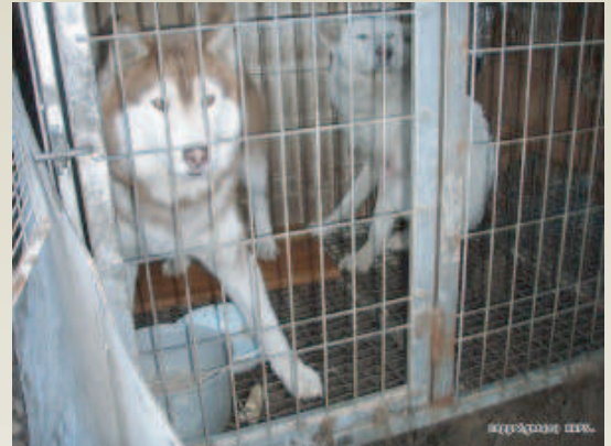
Galvanized welded wire kennel beginning to rust.
